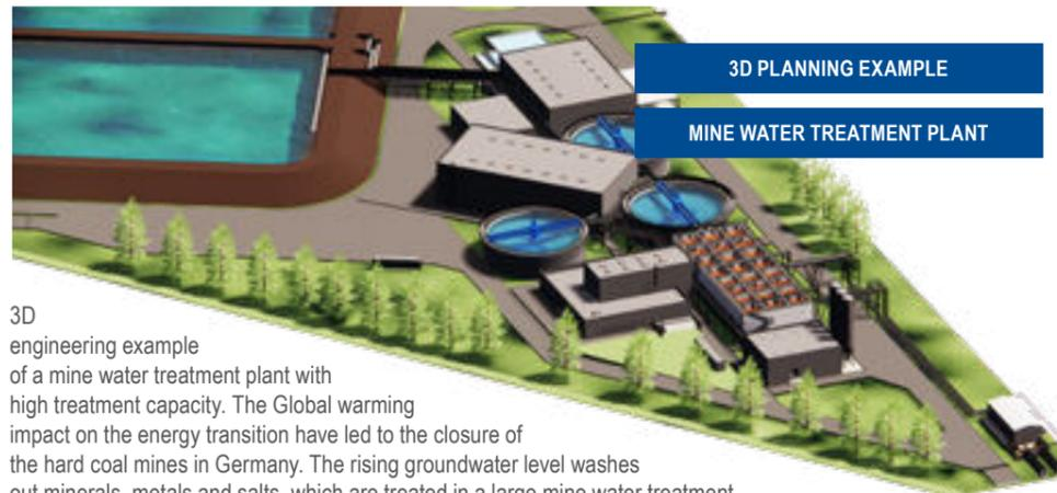
3D engineering example of a mine water treatment plant with high treatment capacity. The Global warming impact on the energy transition have led to the closure of the hard coal mines in Germany. The rising groundwater level washes out minerals, metals and salts, which are treated in a large mine water treatment plant at the RAG site in North Rhine-Westphalia for the discharge into surface waters.
